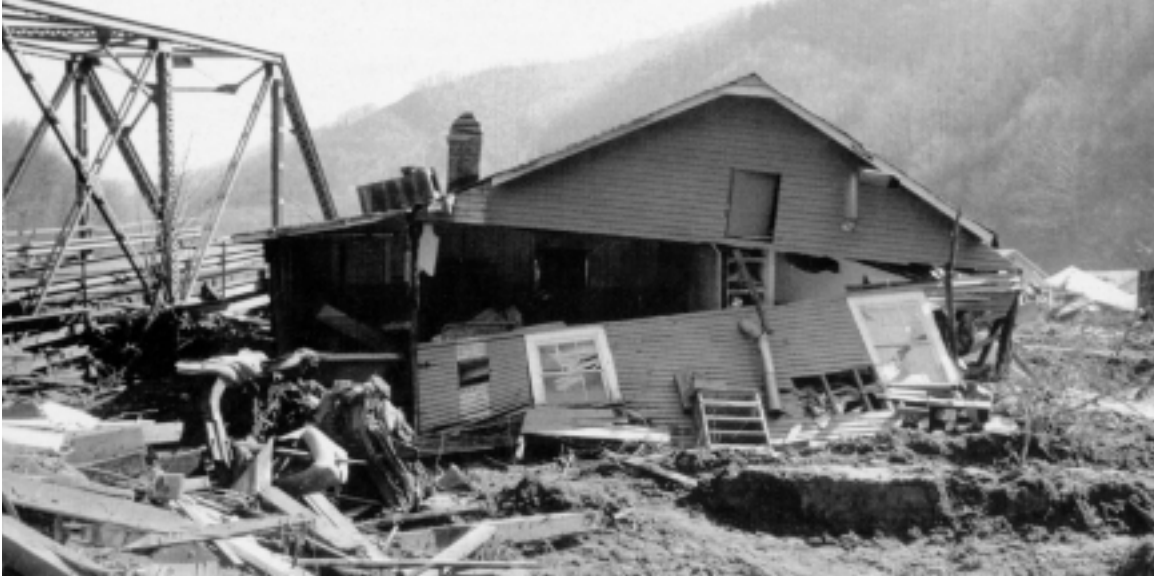
Remnants of homes on Buffalo Creek after the February 26, 1972, disaster. Photo by Jeanne Rasmussen, courtesy of the Archives of Appalachia, East Tennessee State University.
